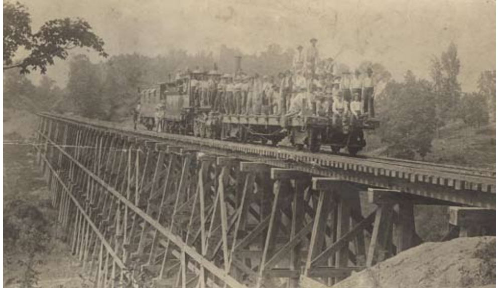
Bear Creek Trestle 1905 - road crew
